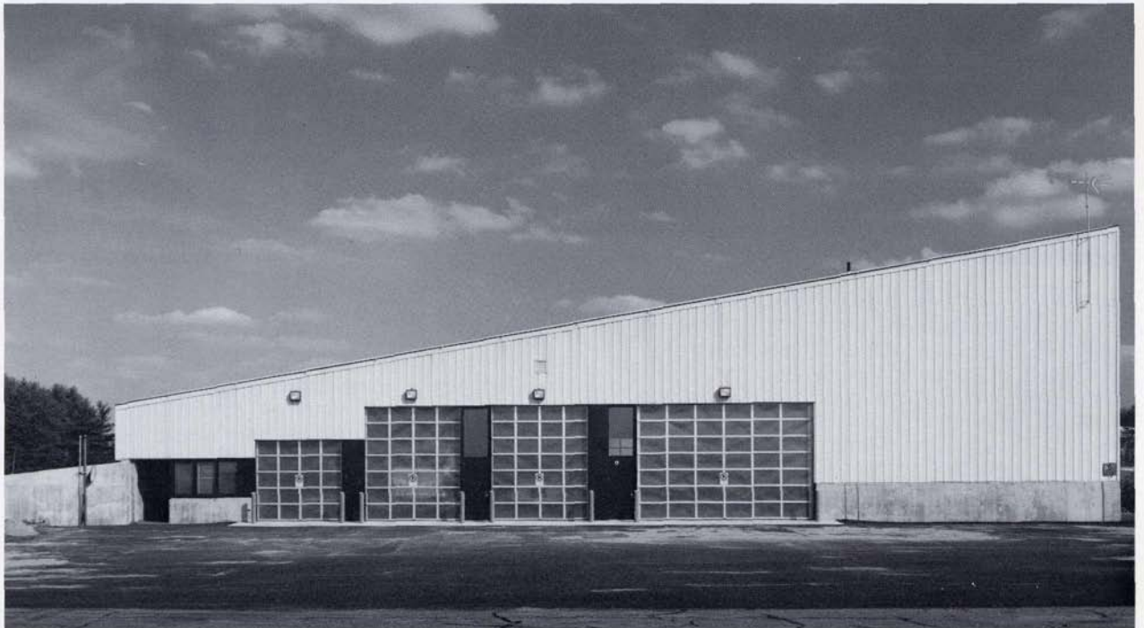
Airport Maintenance Vehicle Garage
